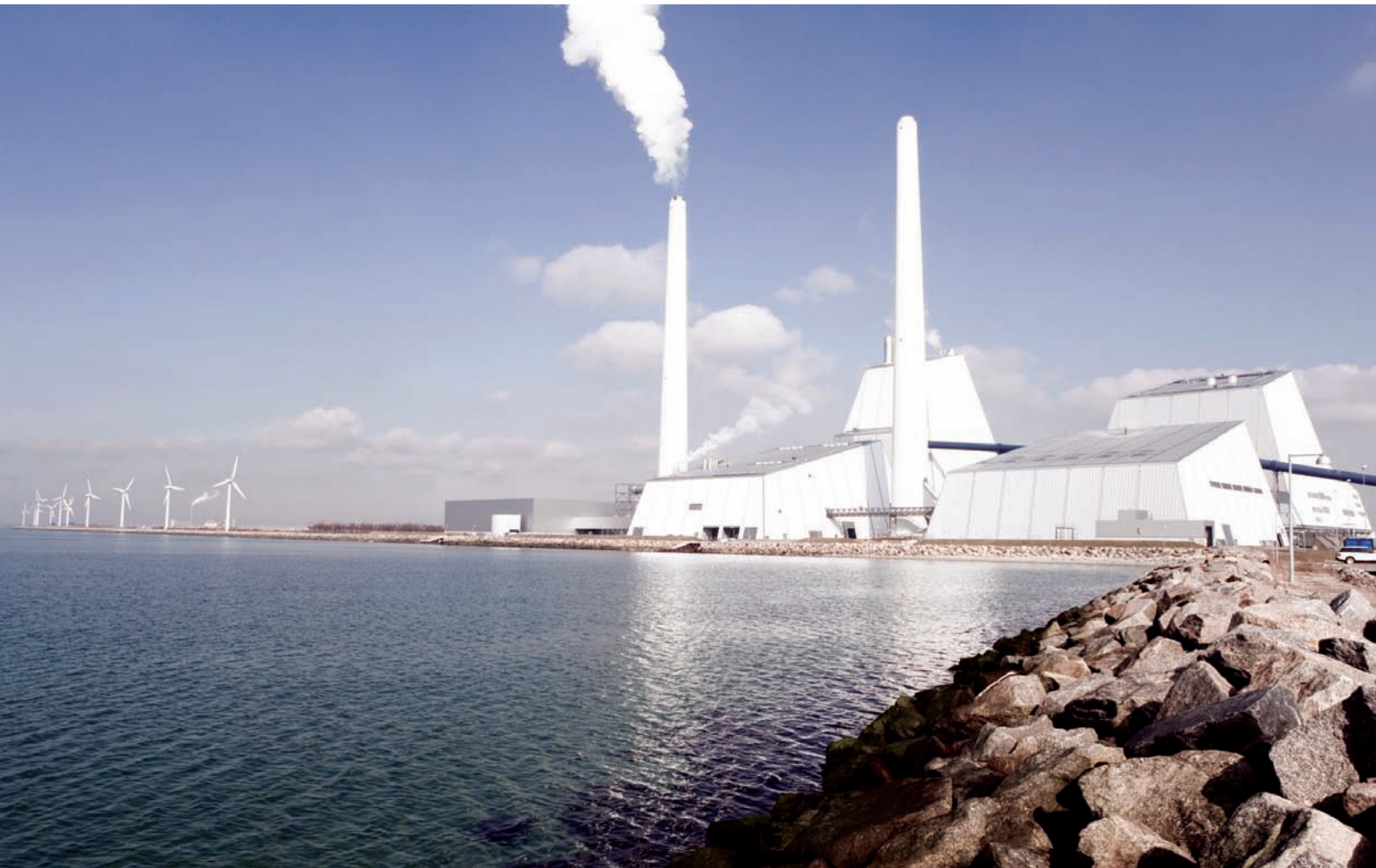
DONG Energy's Avedøre power station, which consists of two units, produces 810 MWe of electricity and 900 MWth of heat and is recognized as one of the world's most flexible power plants
