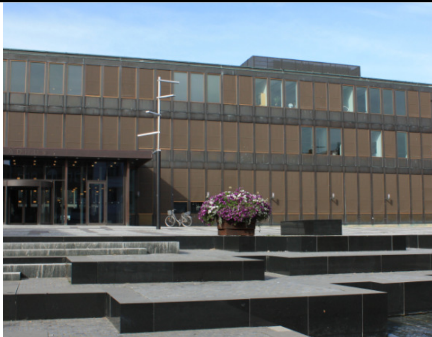
Guards at the service centre in Fredericia receive critical panic alarms on MOTOTRBO radios when employees press their panic buttons.
